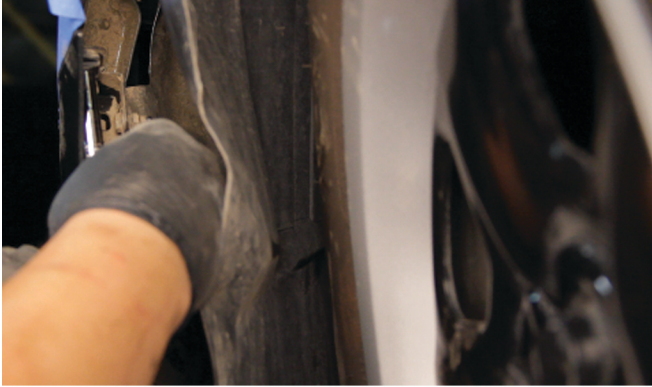
35) Reinstall [1x] 7mm bolts to secure the fascia.
